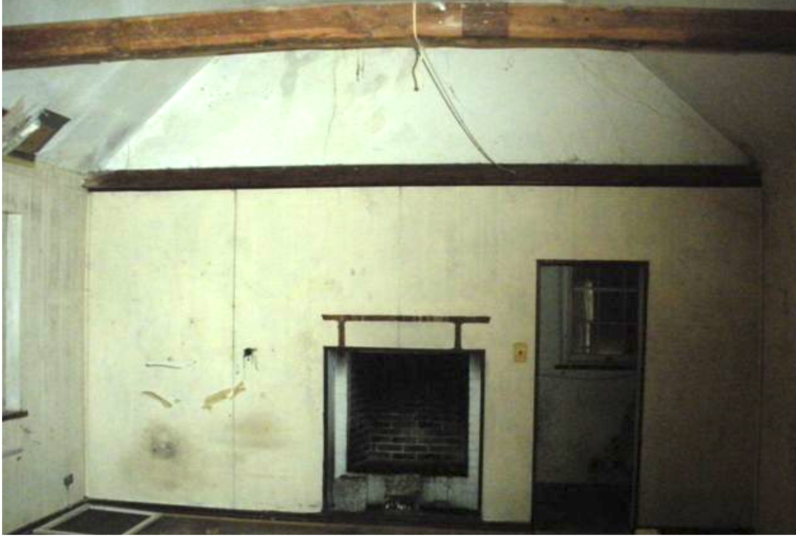
Figure 1.8: Queen of the East retains many of its original interior fittings, including these exposed cedar beams. Courtesy Richard Lowry, 2011.
